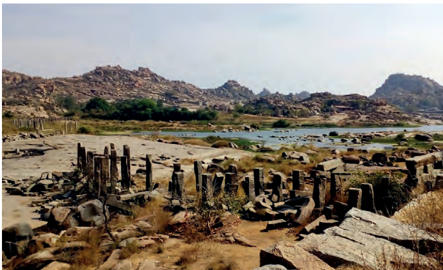
Fig. 1: Ruins of the Vijayanagara period stone bridge across River Tungabhadra with Hampi region's rocky outcrops forming a spectacular background - such popular images of the site overpower the 30-odd living settlements, fields, orchards, markets, and shrines located within the WH boundary. The latter typically do not feature in any popular pictures or promotional materials related to the site.
